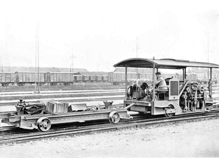
Travels on the rails from Depot to site of operations, under its own power, at a speed of about 25 m. p. h. The Shunting Platform is fitted with wheels and forms a trailer.
